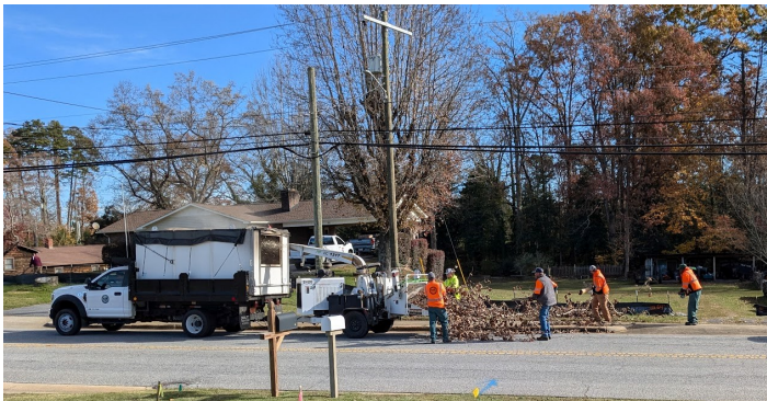
Town of Granite Falls Assisting Caldwell County with Hurricane Helene Debris Pickup
